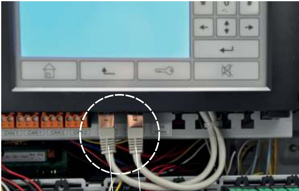
Ethernet Eth1 Ethernet Eth2 E
